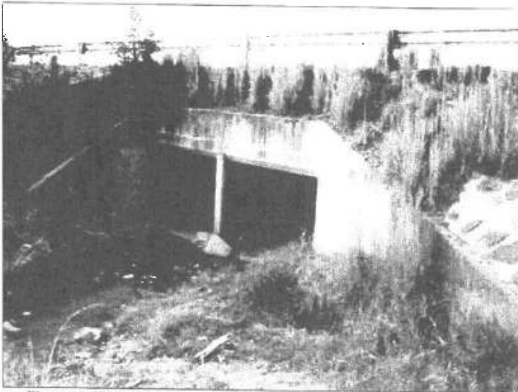
Figure 14: Upstream view of culverts at cross section 220 (River reach A1-2.1)
