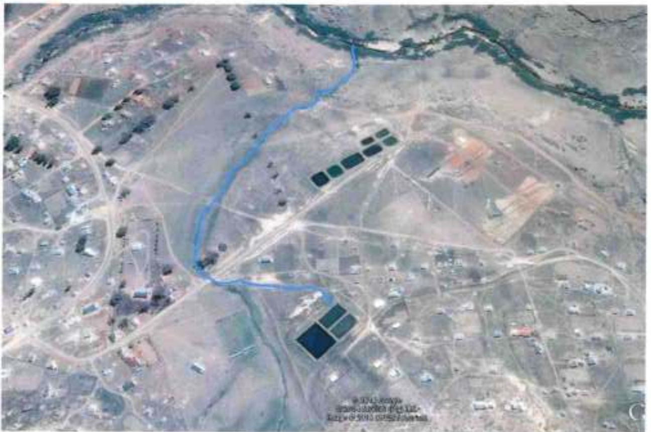
Photo-4: stabilisation pond effluent flowing into the stream, bypassing the 2 nd set of ponds
