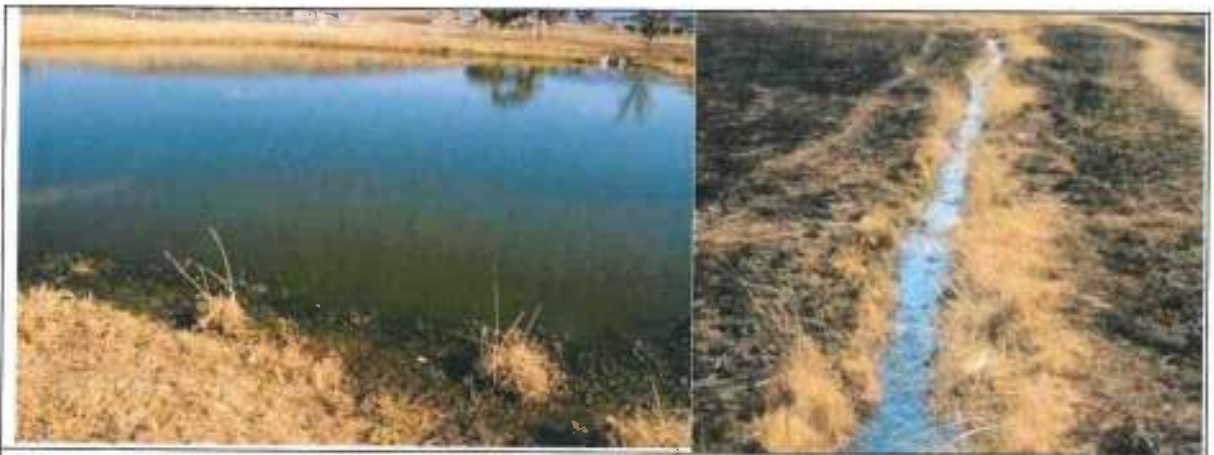
Photo-7: Effluent from set 1 ponds that bypasses the set 2 ponds.
