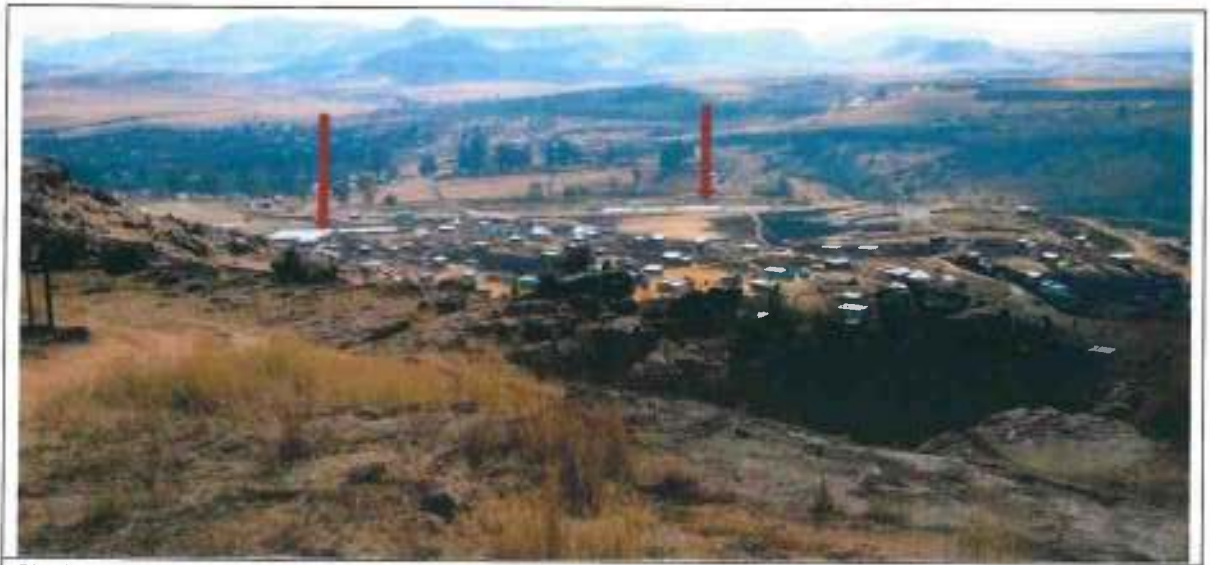
Photo-5: The two sets of oxidation ponds at Mt Fletcher
