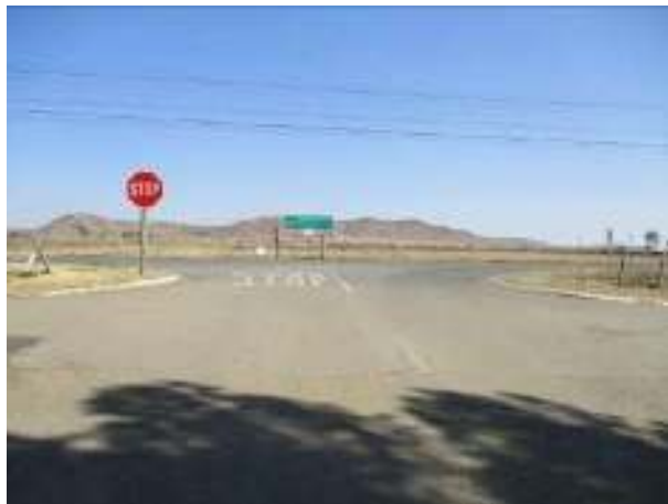
N6/Dan Pienaar Avenue intersection
